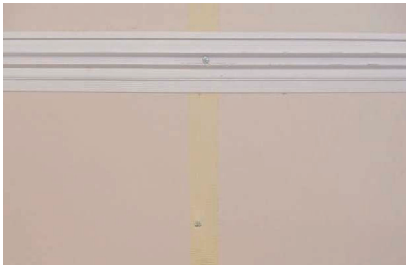
1) Plaster Rail is affixed to wall at a predetermined location prior to finishing.
